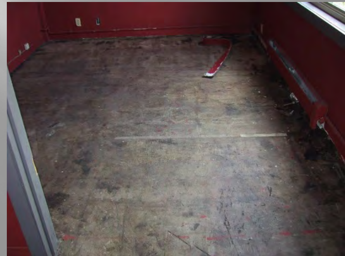
Mastic Removal Always do a mock up!
